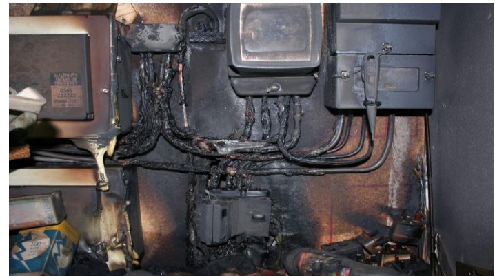
BURNT CABLES IN A JUNCTION BOX
